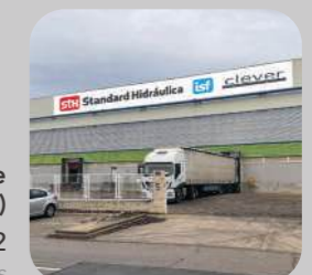
Getafe (Madrid, ES) Superficie 6.500 m2 Facilities / Installations
